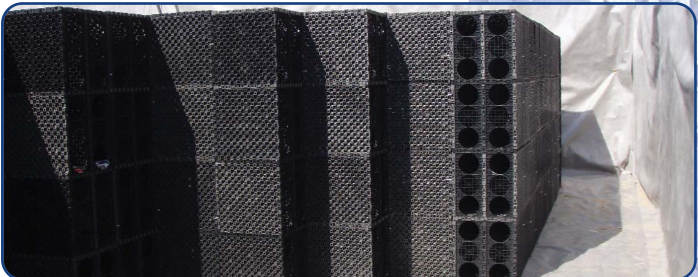
Tank 2mts deep with access channels.
