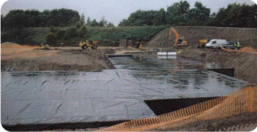
Attenuation Tank under Park and Ride Scheme showing versatility of modular system.
